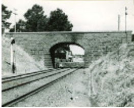
B2094 Road Bridge
