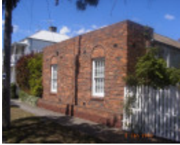
Caledonian Inn (former), Hobsons Bay Heritage Study 2006
