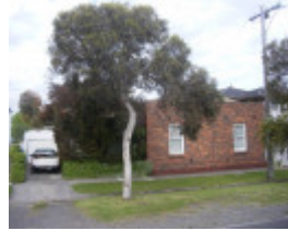
Caledonian Inn (former), Hobsons Bay Heritage Study 2006
