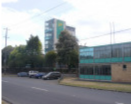
BP Australia Complex and Canary Island Palm, Hobsons Bay Heritage Study 2006
