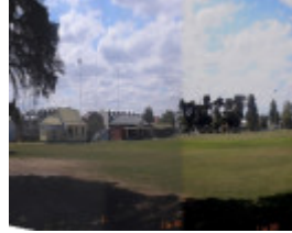
House at 27 Esplanade WILLIAMSTOWN, Hobsons Bay Heritage Study 2006 - overall view looking to the north-west from the Esplanade toward the Tennis Pavilion (bottom left)
