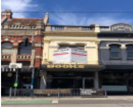
38A Chapel Street, Windsor
