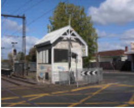
Spotswood Railway Signal Box, Hobsons Bay Heritage Study 2006
