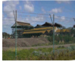
Gilbertsons Meat Processing Complex (Former), Hobsons Bay Heritage Study 2006
