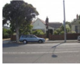
House at 110 Melbourne Road WILLIAMSTOWN, Hobsons Bay Heritage Study 2006
