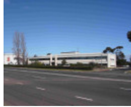
Standard Vacuum Refining Co. Complex (former), Hobsons Bay Heritage Study 2006 - Administrative building (Pegasus Centre) designed by Stephenson & Turner and constructed c.1955
