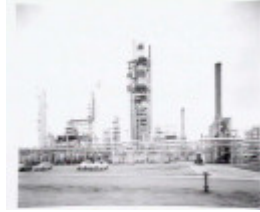
Standard Vacuum Refining Co. Complex (former), Hobsons Bay Heritage Study 2006 - c.1955 view showing Thermofor Catalytic Cracker in centre.
