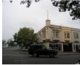
Craigantina, Hobsons Bay Heritage Study 2006
