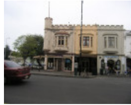
Craigantina, Hobsons Bay Heritage Study 2006
