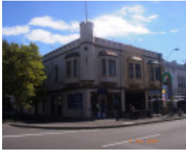
Craigantina, Hobsons Bay Heritage Study 2006
