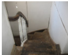
Watford Cottage Avoca 1 Nov 2008 mz Staircase 02
