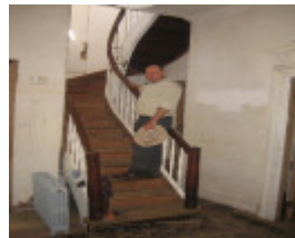
Watford Cottage Avoca 1 Nov 2008 mz Staircase 01
