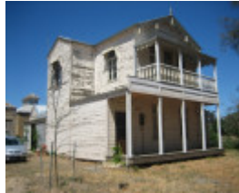
Watford Cottage Avoca 1 Nov 2008 mz Front and North Elevations
