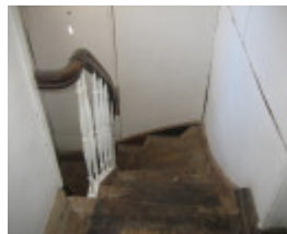
Watford Cottage Avoca 1 Nov 2008 mz Staircase 02
