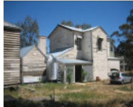
Watford Cottage Avoca 1 Nov 2008 mz North and Rear Elevations
