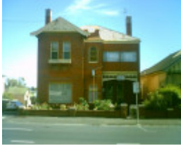
6 Aberdeen Street, Geelong West
