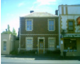
34 Aberdeen Street, Geelong West
