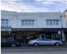
119-125 Wattletree Road, Malvern
