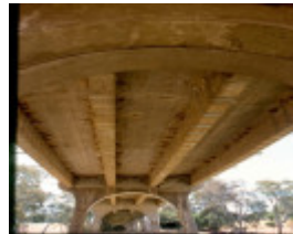
H01986 janevale bridge underside from s jan02
