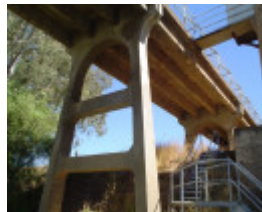
h01986 janevale bridge over loddon river laanecoorie stairs underneath she project 2004
