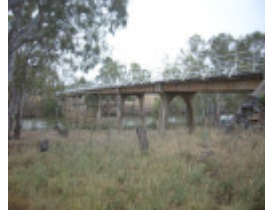
JANEVALE BRIDGE OVER THE LODDON RIVER SOHE 2008
