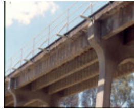
H01986 janevale bridge from sw girders jan02
