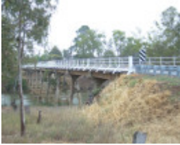
JANEVALE BRIDGE OVER THE LODDON RIVER SOHE 2008
