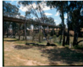
H01986 janevale bridge from se jan02
