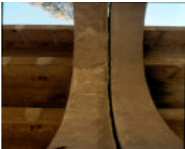
H01986 janevale bridge underside expansion joint jan02
