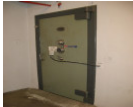
Former Commonwealth Bank Bourke St_Oct 2010
