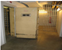
Former Commonwealth Bank Bourke St_Oct 2010
