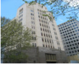
Former Commonwealth Bank Bourke St_Oct 2010
