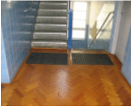
2010_Oct_1_Commonwealth Bank_Melb_site_visit_kj (50).jpg
