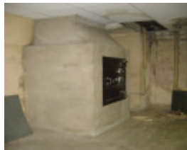
Former Commonwealth Bank Bourke St_Oct 2010
