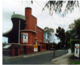
1 glenferrie oval grandstand linda crescent hawthorn side view
