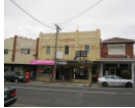
Centenary Hall Waverley Road
