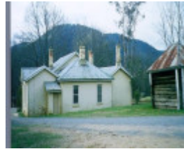
bright courthouse lockup
