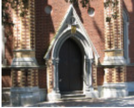
FORMER CONGREGATIONAL CHURCH SOHE 2008
