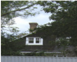
spurling house black street brighton side view sept1999
