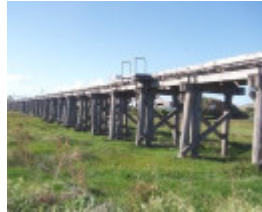
1604 Dennington Railway Bridge
