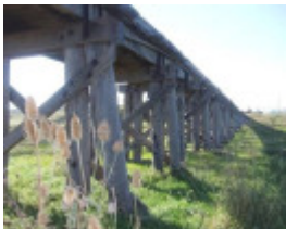
1604 Dennington Railway Bridge2
