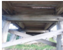
1604 Dennington Railway Bridge3
