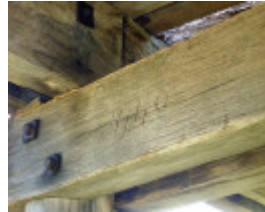
RAILWAY BRIDGE SOHE 2008
