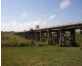
RAILWAY BRIDGE SOHE 2008
