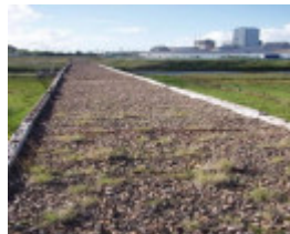
1604 Dennington Railway Bridge4
