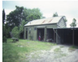
kiora south road brighton stables nov1985
