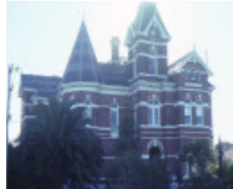
kiora south road brighton front view jun1981
