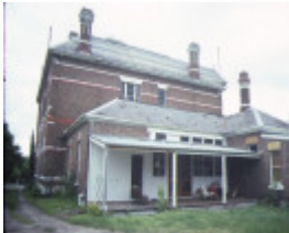
kiora south road brighton rear view nov1985
