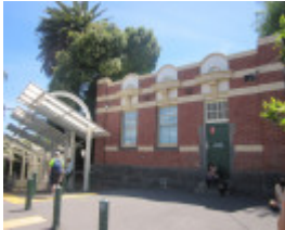
Essendon Railway Complex (Russell Street Entrance).JPG
