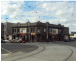
Former Railway Hotel
