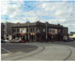
Former Railway Hotel
