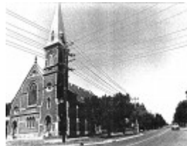
Former Golden Square Precinct 10 - Panton Street Church.jpg
