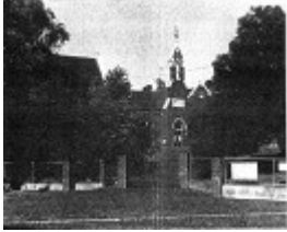
Garvel Hill School, the focal point of the precinct
