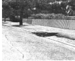
Stone gutters and timber crossovers are now rare in the area but once were universal: Pitt Street.
