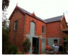
Stables 14 Sorrett Avenue
