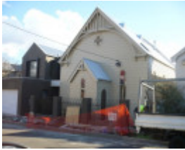
St James' Anglican Church (Former) 2012
