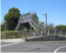
Eglinton Street Pedestrian Bridge.JPG
