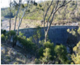
Lower Stony Creek Dam Wall.jpg
