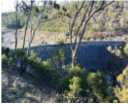
Lower Stony Creek Dam Wall.jpg
