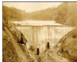
The outer face of the dam wall during construction 1873 (Image Barwon Water).gif
