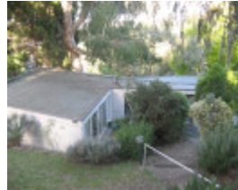
Snelleman House former carport
