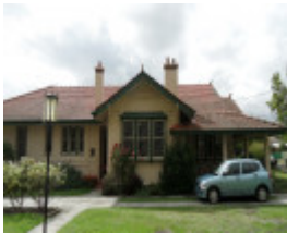
St Mary's Presbytery, west side
