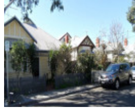
Edwardian timber villas, Benson Street
