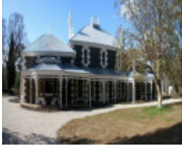
Eynesbury Homestead - Eynesbury Road EYNESBURY, MELTON SHIRE
