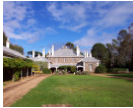
Rear of homestead - workers quarters
