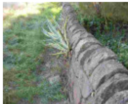
Dry Stone Wall M176 - HaHa Wall
