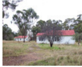
Prefabricated Myer houses
