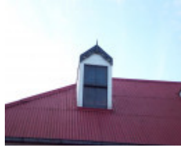
Dormer window (front elevation of Homestead)
