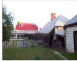
Exford Homestead - rear elevation
