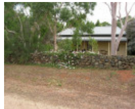
Dry Stone Wall L156
