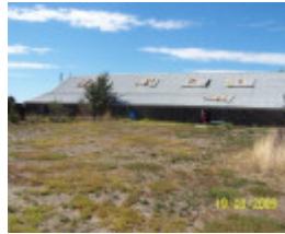
Deanside Woolshed Complex - 96-103 Reed Court ROCKBANK, MELTON SHIRE
