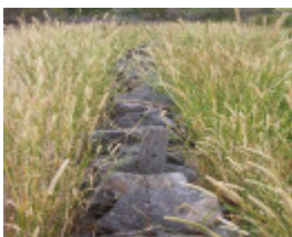
Deanside - Dry Stone Wall
