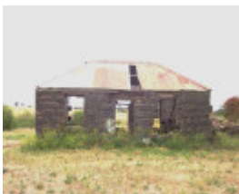
Deanside - Cook's House
