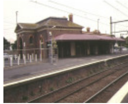
1 brighton beach railway station platform jan1995
