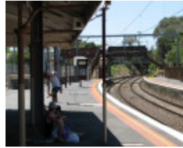
BRIGHTON BEACH RAILWAY STATION SOHE 2008
