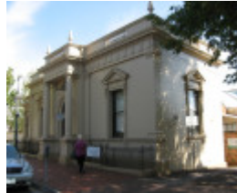
Mechanics Institute_Hamilton_1872 facade_KJ_April 09
