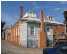
Mechanics Institute_Hamilton_rear view with 1903 additions_KJ_April 09
