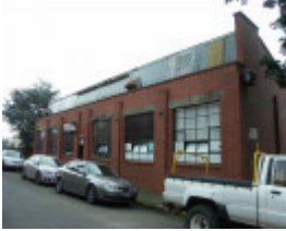
Factory, south (main) elevation
