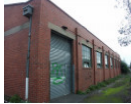
Factory, north (rear) elevation
