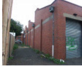
Factory, east (side) elevation
