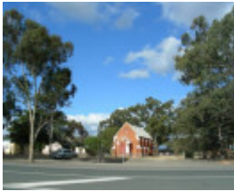
St Stephen's Anglican Church - front aspect from road 2008
