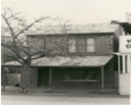
B2634 Old Brick Shop
