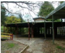
Before Photograph - Reference F3896 2014
