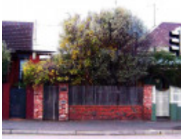
RICHMOND BURNLEY STREET 105.jpg
