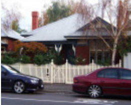
RICHMOND BURNLEY STREET 116.jpg
