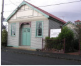
9-13 Clarence Street, Geelong West
