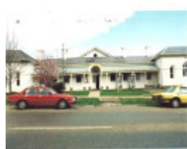
Alexandra court house
