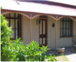
IRON HOUSE SOHE 2008
