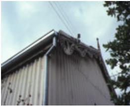
iron house brunswick road brunswick side view aug1980
